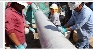
**The A+ Wrap**<sup>™</sup> **System** is a high-strength, water-activated fiberglass composite pre-impregnated with moisture cured polyurethane resin. It is designed for simplification of installation for restoring the structural strength of degraded pipe with varying geometries. It is also able to be used for pressure containment under certain circumstances.
