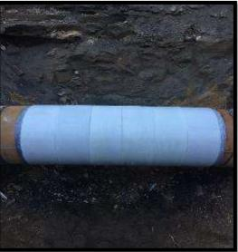
12. Top coat the repair if required (a top coat is always recommended over our repair systems).
