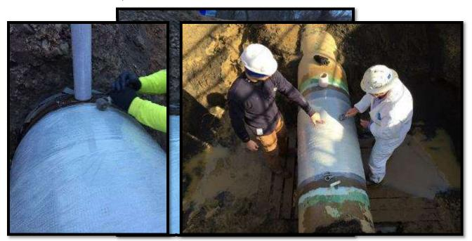
10. Immediately perforate the constrictor wrap to allow for out-gassing and de-bulking.
