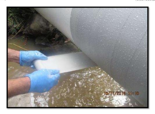
9. Immediately upon completing the installation (or at a hold point), wrap 4-6 layers of constrictor wrap.
