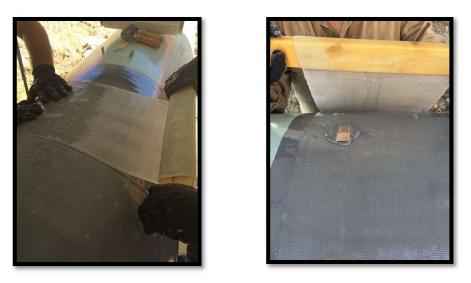
7. Begin application of the Atlas<sup>™</sup> material. Mix Epoxy Resin kits (A&B) and impregnate necessary lengths of carbon fabric.
