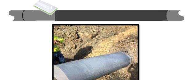
6. Mix an Epoxy Resin kit (Parts A&B) for approximately 1 minute and apply the resin to the fiberglass fabric until it is saturated. Excess resin can be scraped off using the blue squeegee. Apply a fiberglass layer to the repair zone. Install ILI Marker<sup>™</sup> system if applicable.
