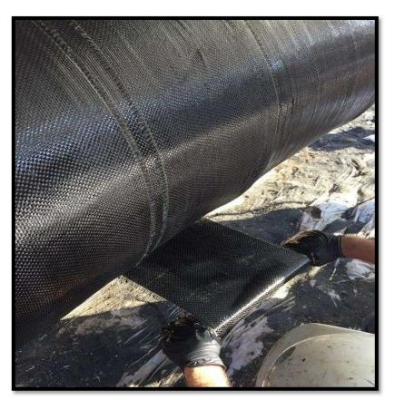
9. Immediately upon completing the installation (or at a hold point), wrap 4-6 layers of constrictor wrap.
