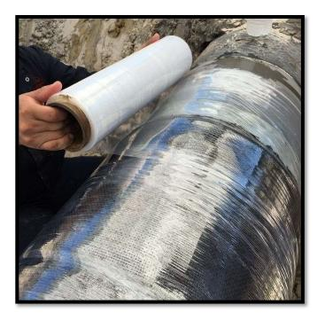
10. Immediately perforate the constrictor wrap to allow for de-bulking.
