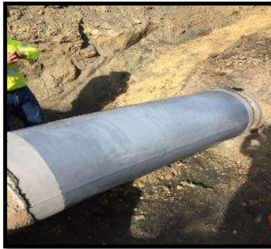
6. Mix an Epoxy Resin kit (Parts A&B) for approximately 1 minute and apply the resin to the fiberglass fabric until it is saturated. Excess resin can be scraped off using the blue squeegee. Apply a fiberglass layer to the repair zone. Install ILI Marker™ system if applicable.
