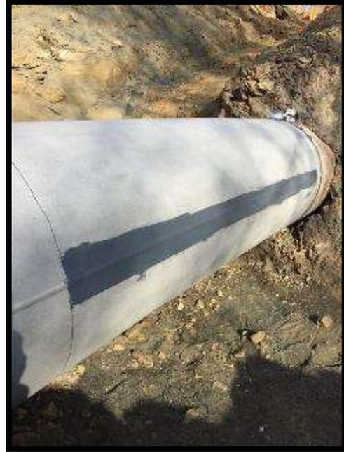
4. Mix and apply specified Load Transfer Filler materials over all defect and tented areas (i.e. welds), trying to return the pipe to a near-net profile. Smooth to pipe as needed.
