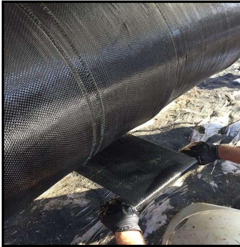
9. Immediately upon completing the installation (or at a hold point), wrap 4-6 layers of constrictor wrap.
