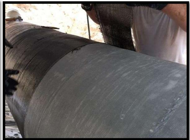
8. Continue wrapping per installation method. Once two layers have been achieved, ensure that constant, uniform tension is applied to the roll.
