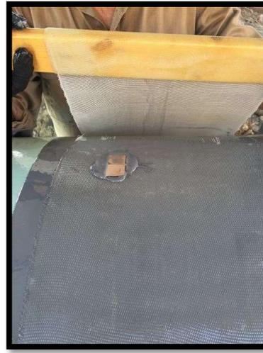
7. Begin application of the Atlas™ material. Mix Epoxy Resin kits (A&B) and impregnate necessary lengths of carbon fabric.
