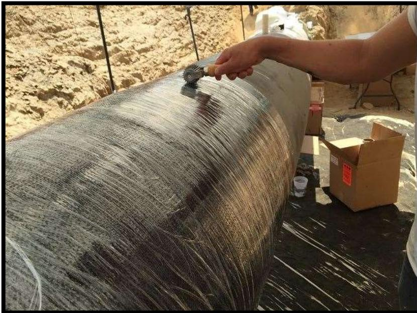
11. Allow the repair to cure for a minimum of 2 hours, before removing constrictor wrap.
