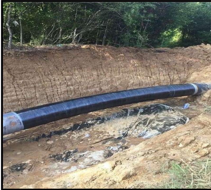
12. Top coat the repair if required (a top coat is always recommended over our repair systems).
