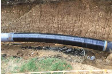
**Atlas™** is a high strength, high stiffness carbon fiber solution for on-site repair of piping structures. Atlas™ is designed for repairs requiring strain reduction due to dynamic loading conditions
