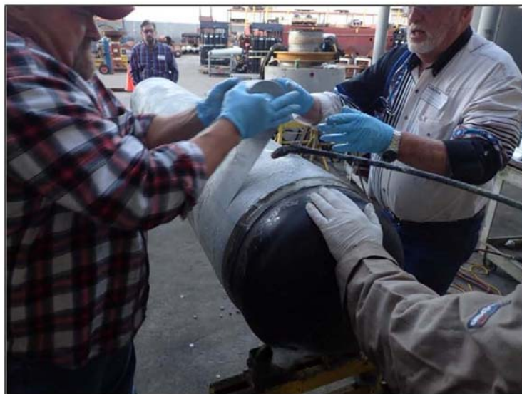
Figure 6: Installation of the Western Specialties ComposiSleeve System
