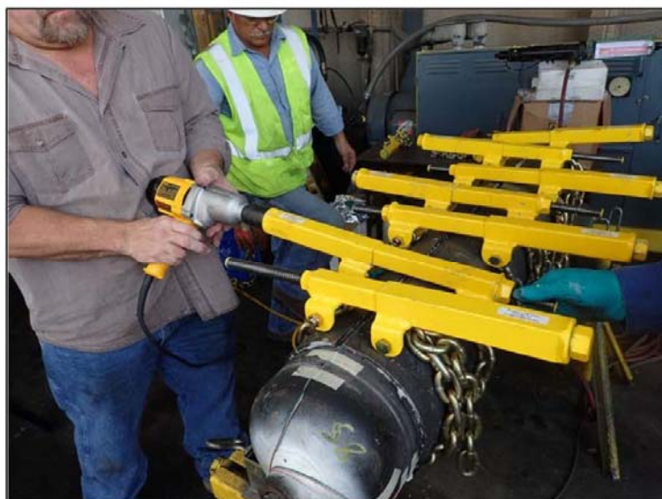
Figure 5: Installation of the Western Specialties ComposiSleeve
