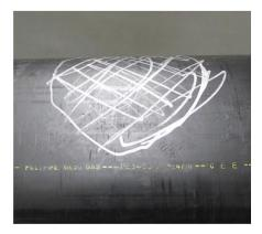
**Step 2:** Using the scraping tool, remove outer layer of pipe in order to reach virgin material.
