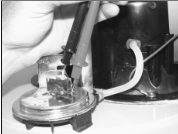
Blocked Exhaust Switch FPSH 260 Series
